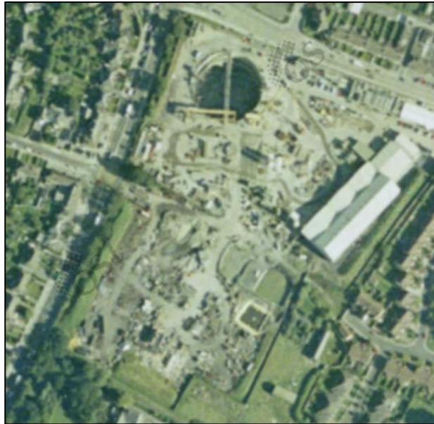
Figure 14-1 2005 Aerial photograph of the site showing the level of disturbance
